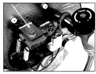
If fitted, mixing valve also has an air relief screw M5, which shall be opened. (Picture 7)
